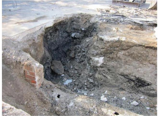
Fig. 15 - Identified TPH-impacted soil near to passive soil gas sampler GS19.
