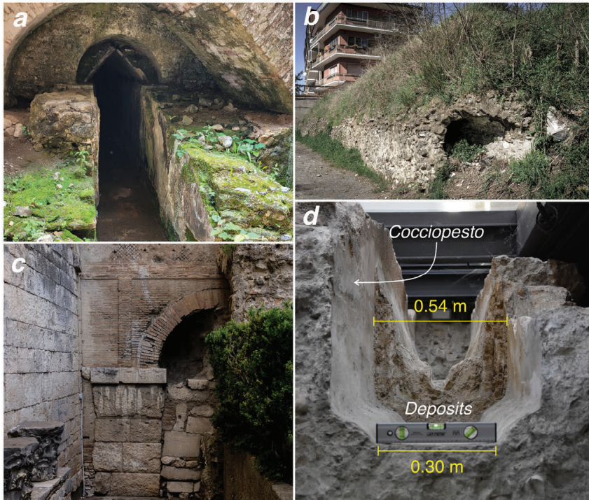
Fig. 3 - Sannitico Aqueduct (1 century B.D.): a) beginning of the aqueduct tunnel near the Urcioli Spring of the Serino group (Caput Aquae); b) ruins located along Avellino Street in Benevento city; c) the opus reticulatum highlights the main channel remain under Rocca dei Rettori building; d) detail of the main channel inside Rocca dei Rettori building.
