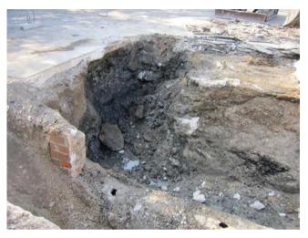
Fig. 15 - Identified TPH-impacted soil near to passive soil gas sampler GS19.
